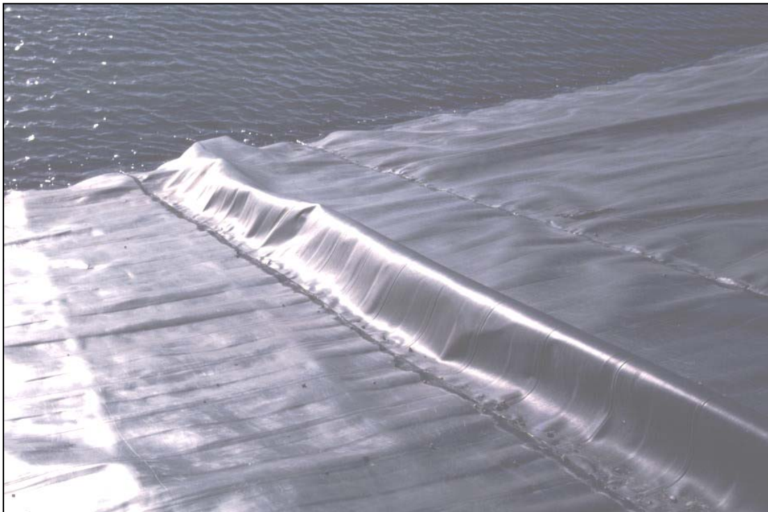
Fig. 9: Compensation panel. [Photo J.P. Giroud]
