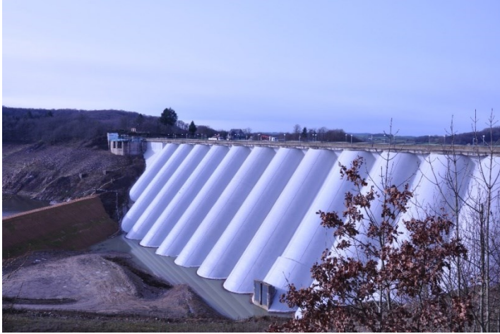
Figure 19. Pannecière Dam in France [Courtesy Carpi].
