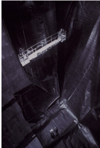
Figure 13. The cavity during geomembrane liner installation.
