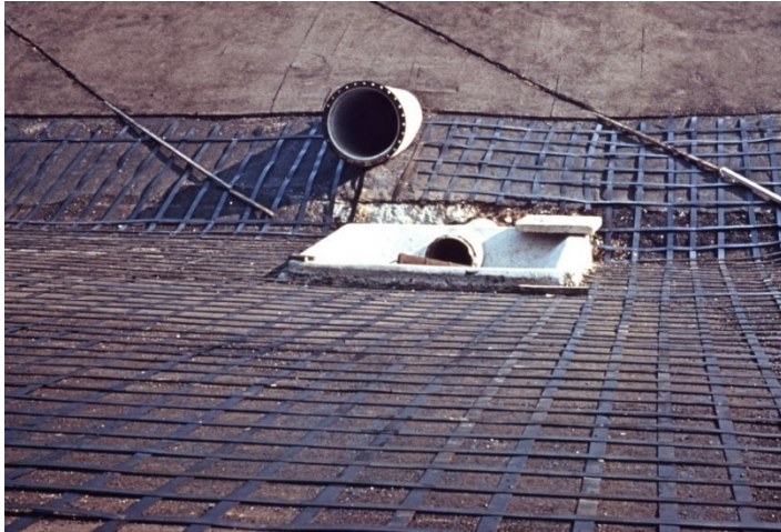
Figure 7. Steel reinforcement used in the secondary liner made of bituminous concrete.
